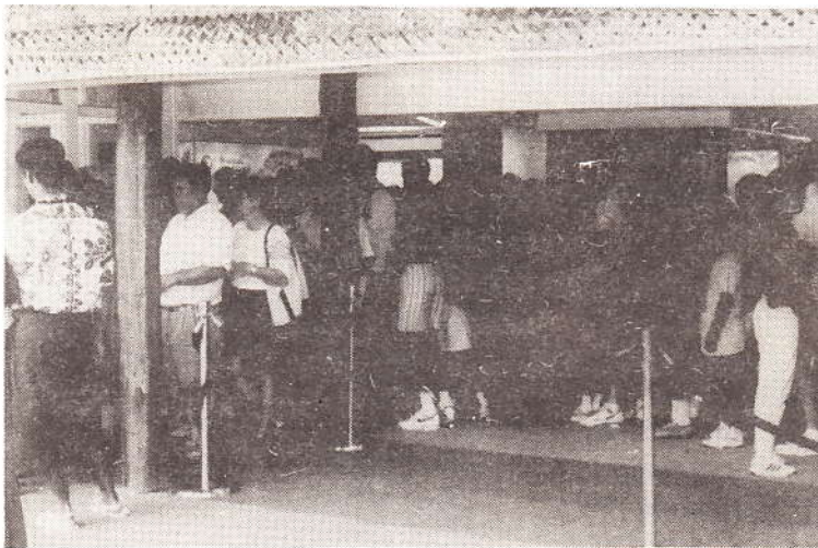
Guests line up in new renovated entrance
