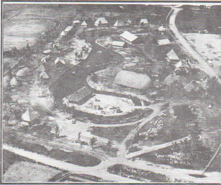
1963 - Construction of the Center is well underway by labor missionaries.
