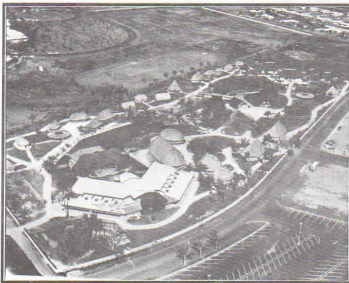
1963 - Most construction is now complete and Center is open for business, Notice the difference that just a few months can make.
