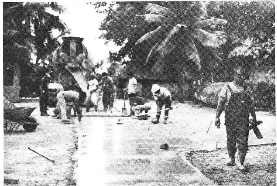
Workmen follow along behind cement truck to smooth out new walks in Samoan Village.
