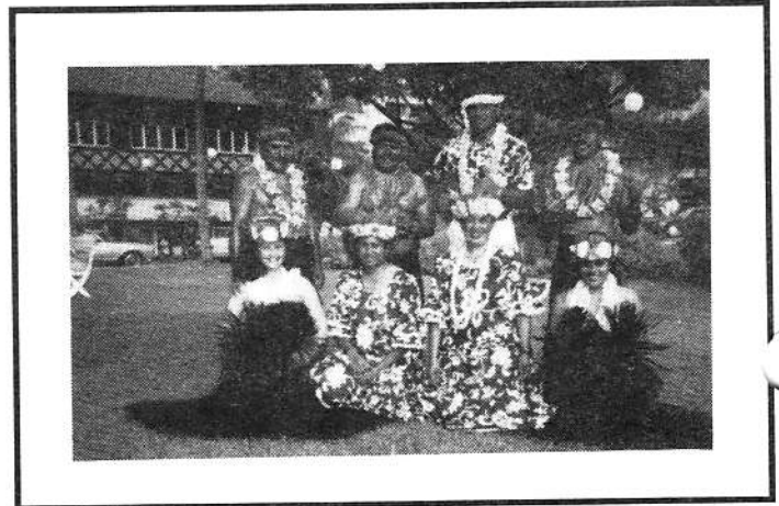
At the Hilton Hawaiian Village Hotel, the Tahiti Village/Village Operations promo group.
